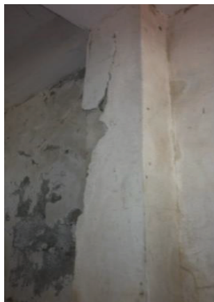
(a) Cracks in the column at corner C4 column (Site No 04- 1 st floor)
