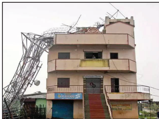
Figure 1 - Failure of a Tower in Chennai in India during Cyclone Phailin in 2013 [2]
