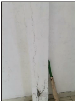
(b) Cracks in the column at C3 column (Site No 04- First Floor)
